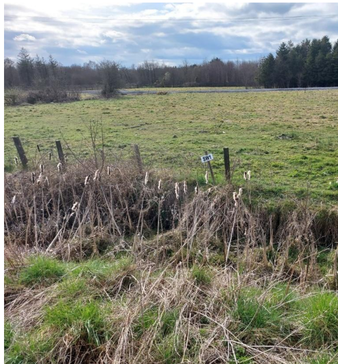
Photo 4: Example of an Operational Phase Settlement Pond
